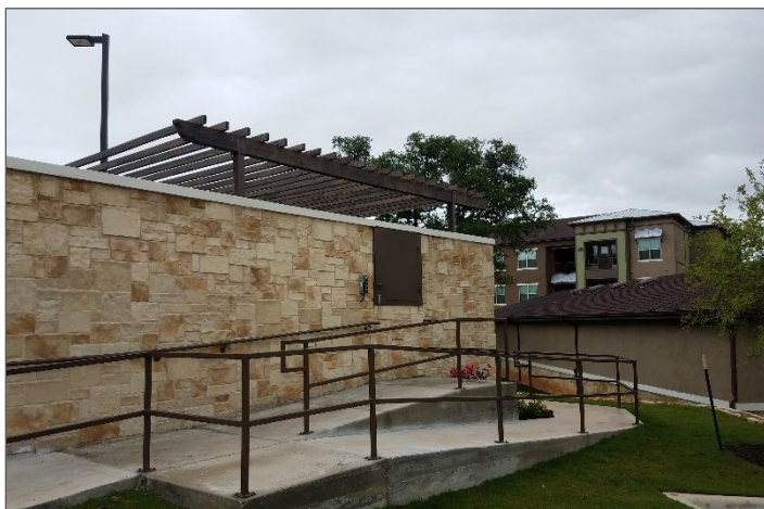
Multifamily compactor enclosure
